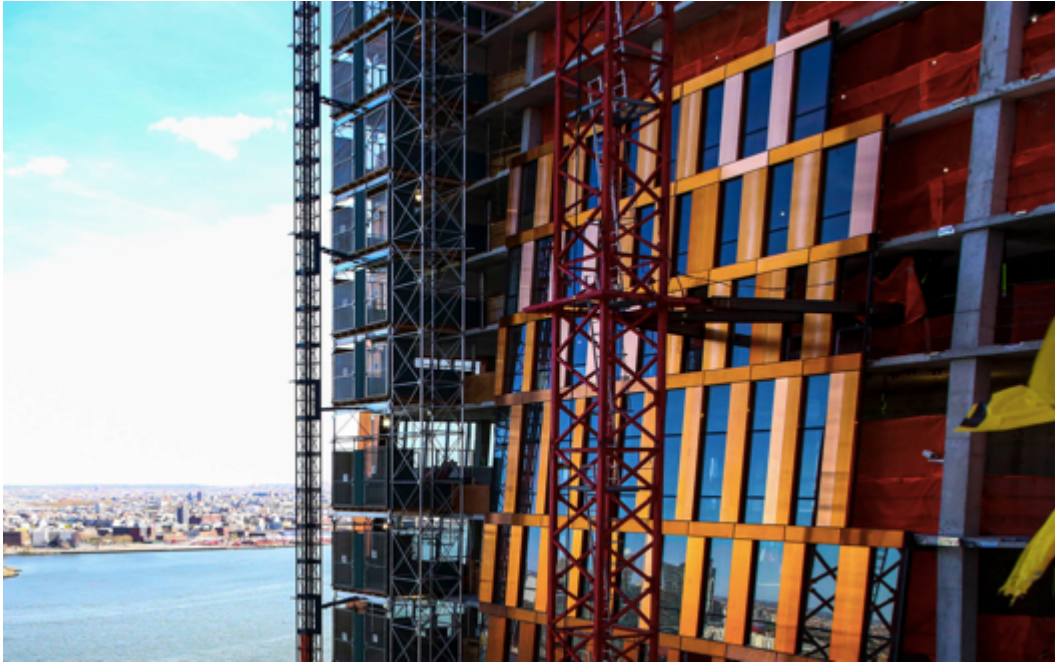
The copper cladding before it ages and turns green. Photographer: Chris Goodney/Bloomberg
