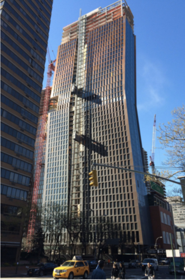
American Copper Buildings under construction.
