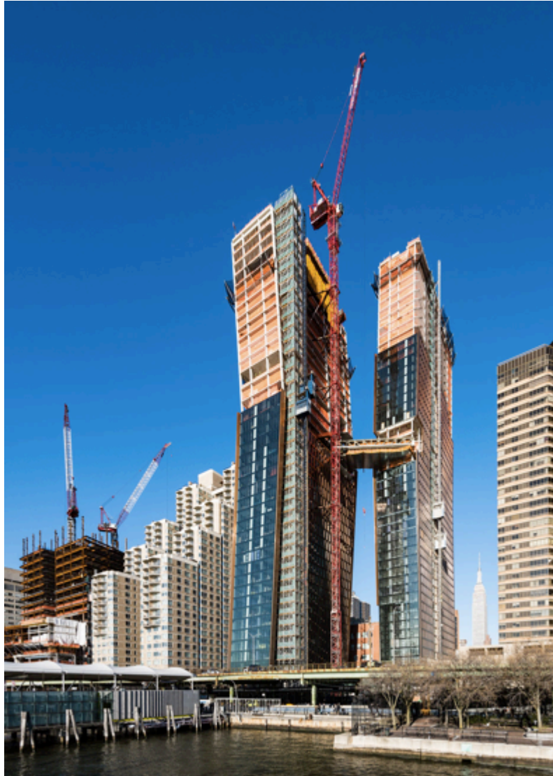
The three-storey skybridge links the towers at floors 27 to 29
