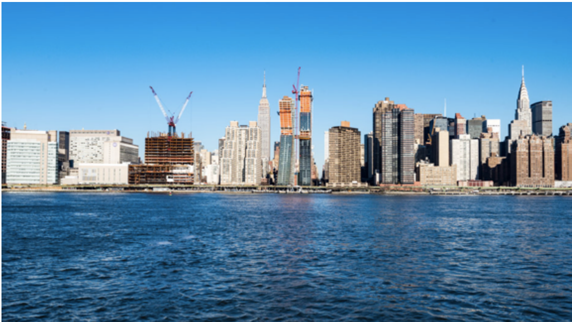
The bendy towers are rising along the East River
