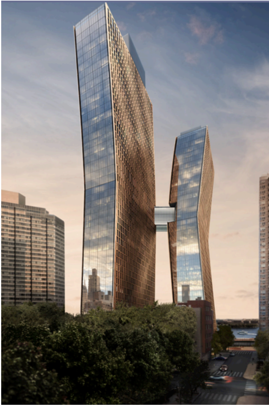
The 41- and 48-storey towers will be linked by a skybridge and clad in copper and glass
