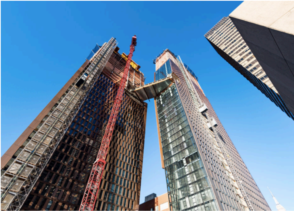
The skybridge is suspended 300 feet above the ground
