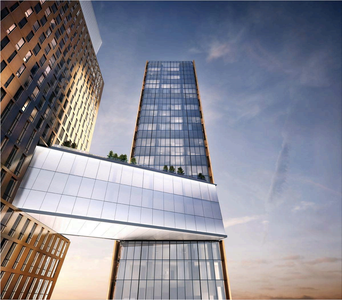
A detail from sky bridge. Image © MARCH
