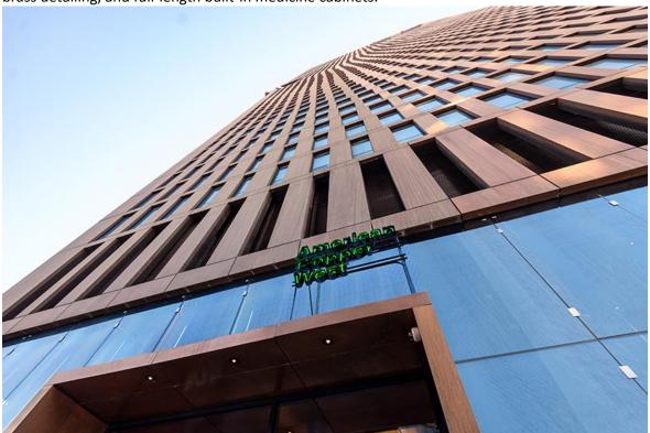
the structure is clad in 4.25 million pounds of raw copper
